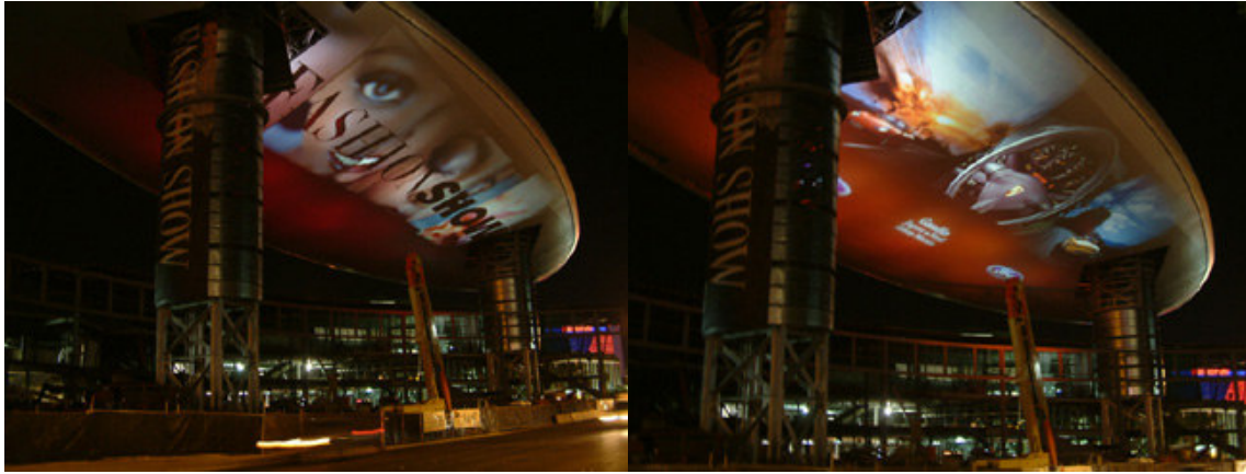
Figure 4. Cloud after cladding installation
